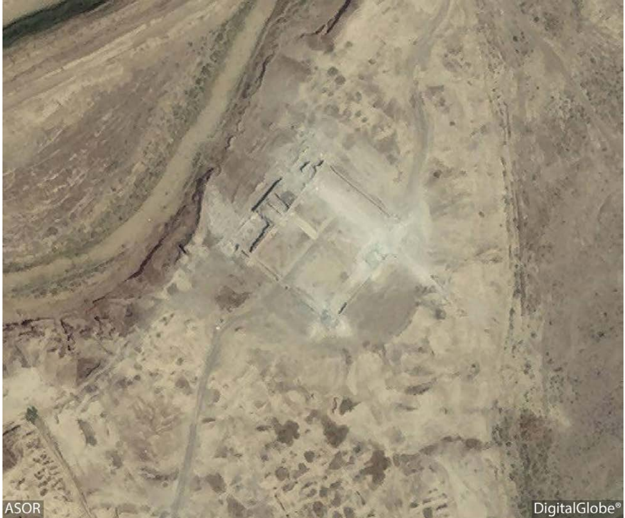
Satellite image showing damage to the Farhan Pasha Palace (Ottoman Barracks) and the area around the Temple of Assur, Assur, Iraq (DigitalGlobe; ASOR CHI; taken June 10, 2015)
