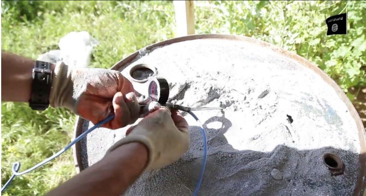
Northwest Palace, Nimrud, Iraq, ISIL militants setting the fuses of the barrel bombs (YouTube; screenshot of video posted by ISIL-associated account, showing the demolition of the Northwest Palace)
