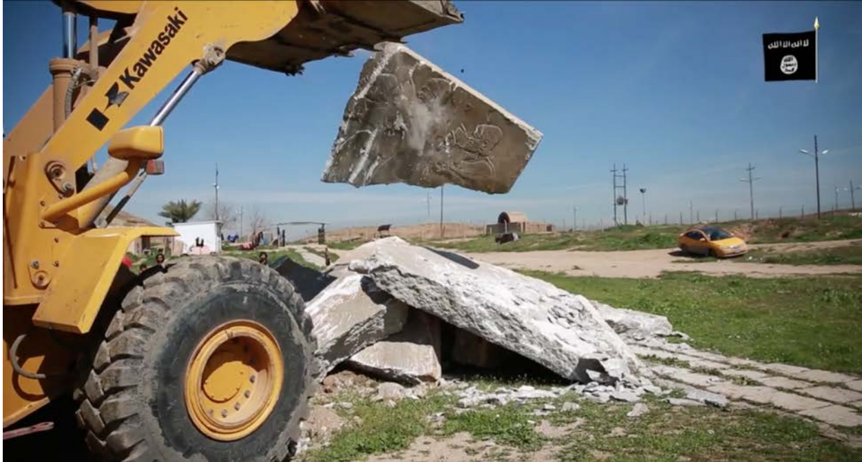
Northwest Palace, Nimrud, Iraq, ISIL militants removing the rubble of the wall relief panels with a bulldozer (YouTube; screenshot of video posted by ISIL-associated account, showing the demolition of the Northwest Palace)
