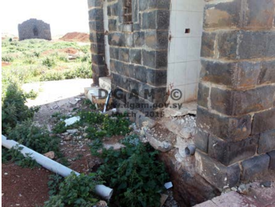
The Ottoman railway buildings north of al-Taiba (DGAM; posted April 11, 2015)
