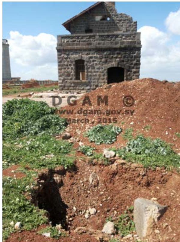
The Ottoman railway buildings north of al-Taiba (DGAM; posted April 11, 2015)
