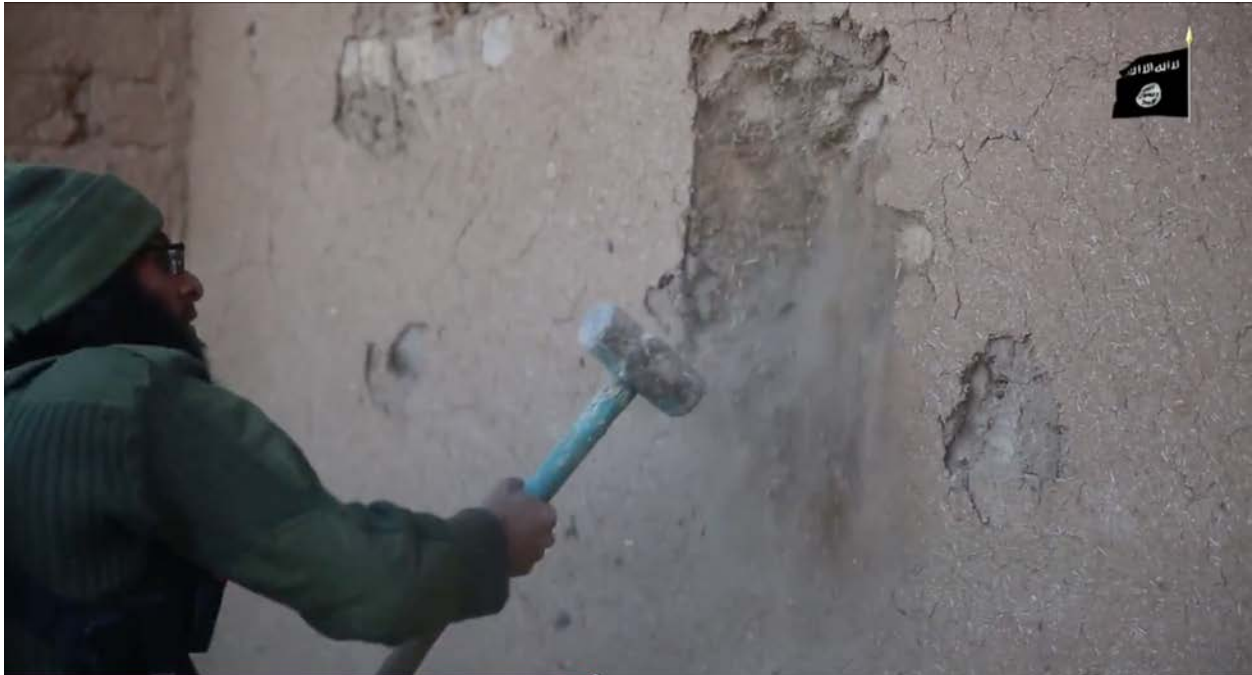
Northwest Palace, Nimrud, Iraq, ISIL militant attacking the site with a sledgehammer (YouTube; screenshot of video posted by ISIL-associated account, showing the demolition of the Northwest Palace)
