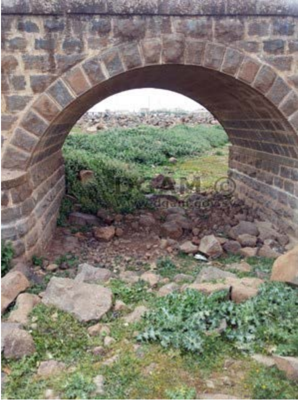
Ottoman railway bridge in al-Taiba (DGAM; posted April 6, 2015)
