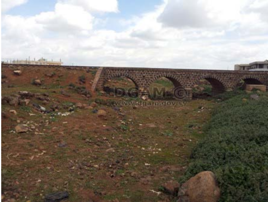
Ottoman railway bridge in al-Taiba (DGAM; posted April 6, 2015)
