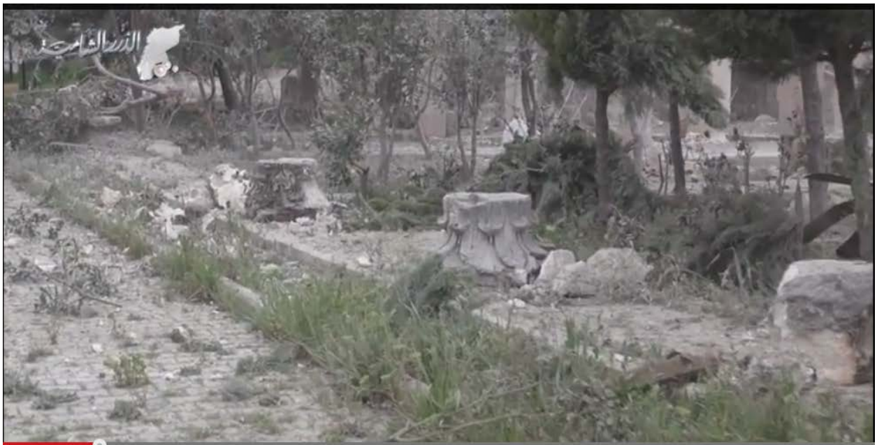
Idlib Museum, damage to the exterior (screenshot from YouTube footage posted by APSA on April 1, 2015)
