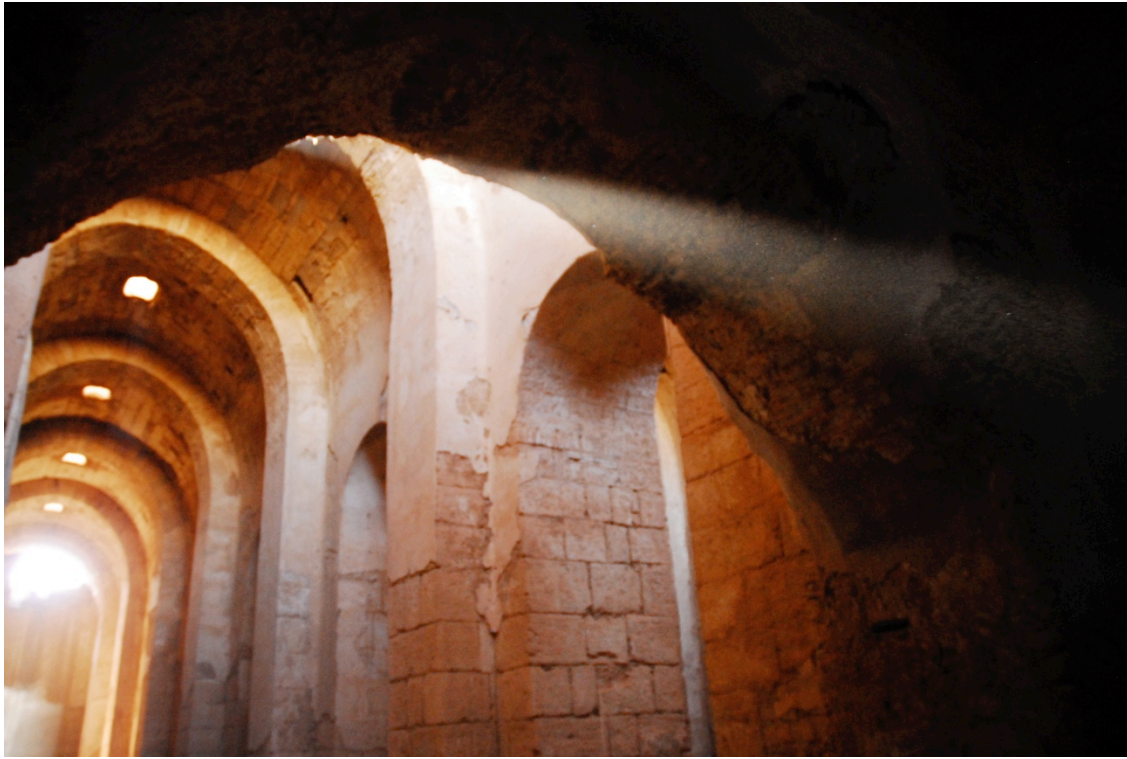
The interior of the cisterns at Resafa (Michael Danti 2010).
