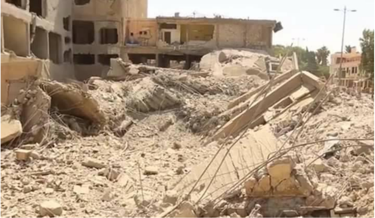
Damage to structures near the Raqqa Museum (Private Facebook Account; June 7, 2017)
