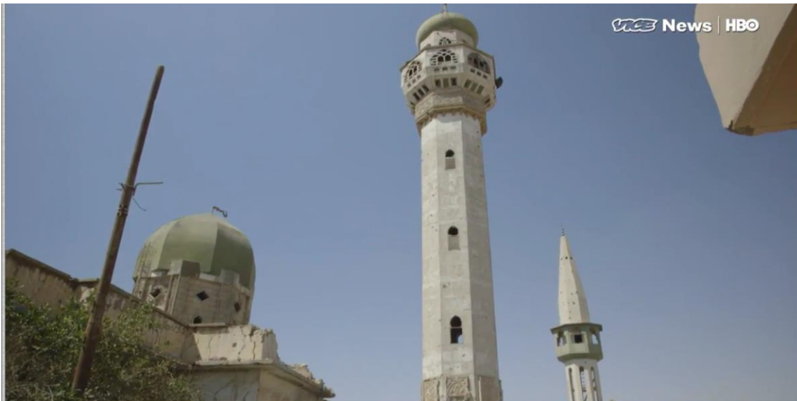
Damage to al-Imam Muhsin Mosque and Minarets (Vice News; June 30, 2017)
