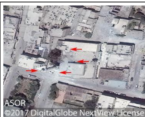
The top of the minaret is broken and there is debris on top of the mosque (DigitalGlobe NextView License; June 17, 2017)
