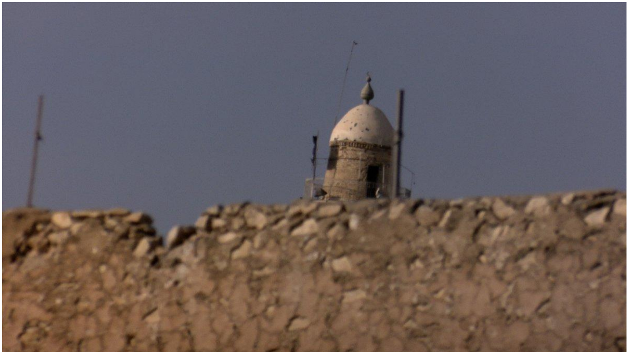
al-Hadba Minaret, including some possible damage to the top of the minaret, hours before its destruction (Feras Kilani; June 22, 2017)
