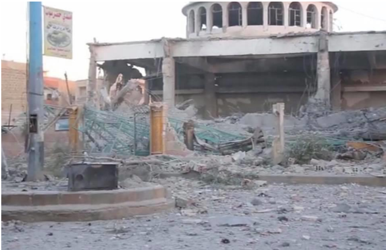
Damage to al-Nur Mosque (RBSS: June 10, 2017)
