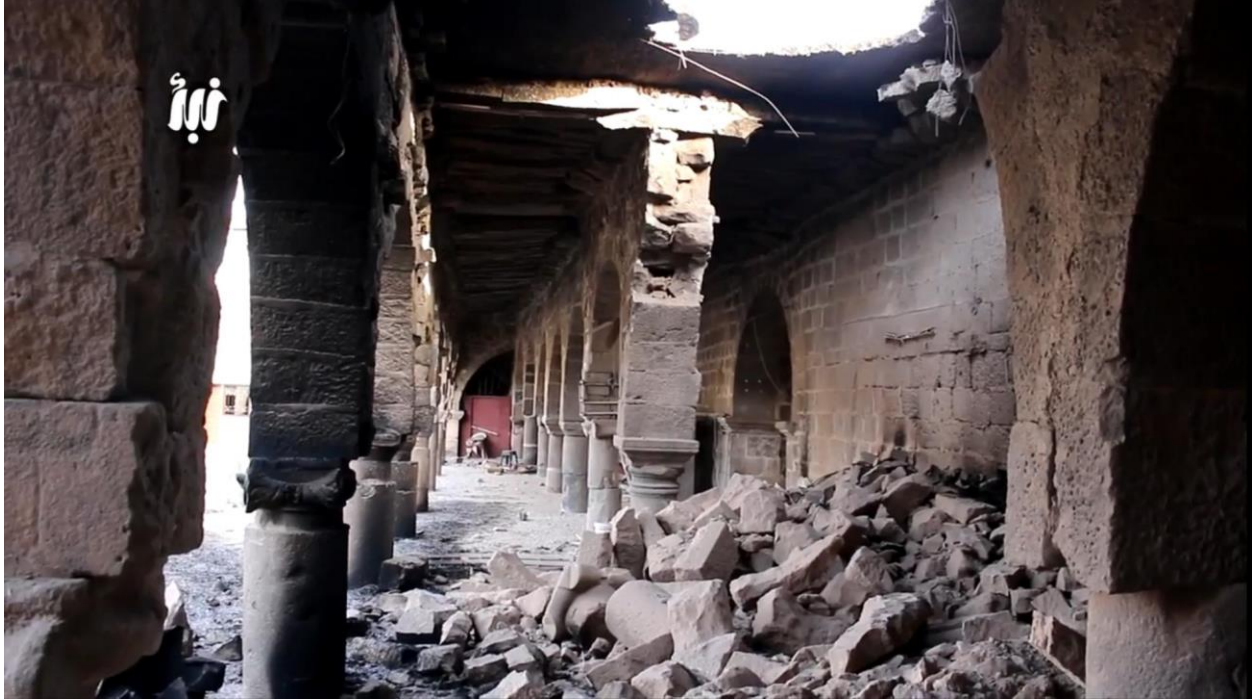
Video still of damage to the portico along the side of the courtyard (Nabaa; June 9, 2017)
