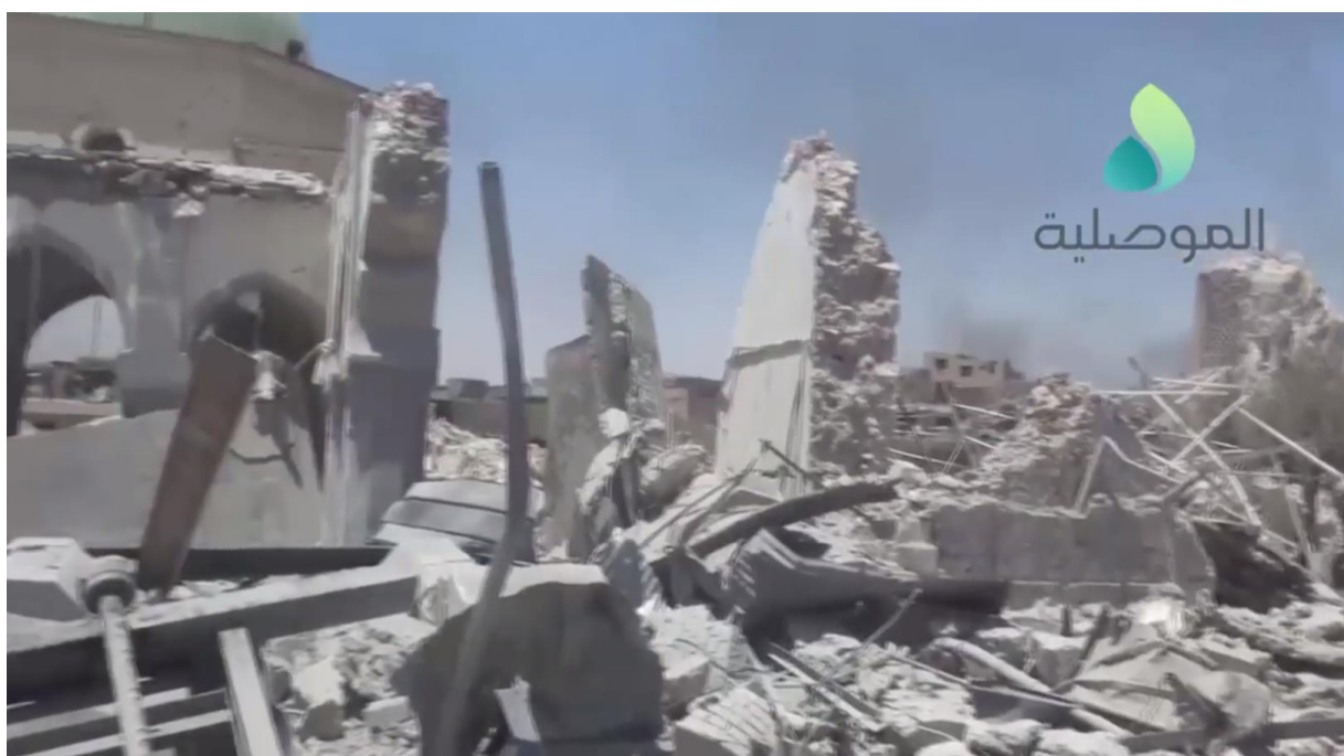
Destruction to al-Nuri al-Kabir Mosque and al-Hadba Minaret (Al Mousliya; June 30, 2017)
