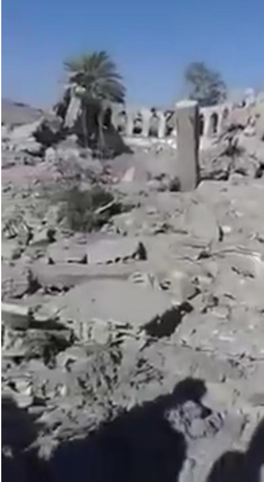
Video still of damage to Zubair bin Awam Mosque (SNHR; June 29, 2017)
