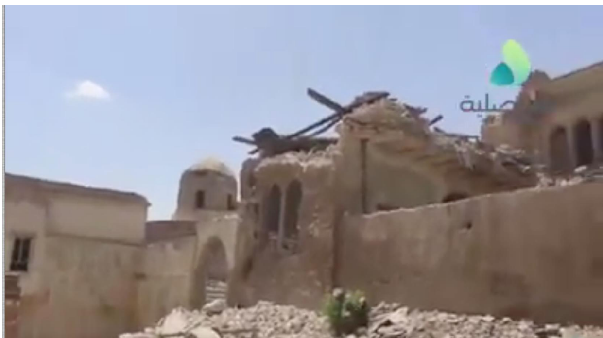
Video still of part of Mar Thomas Church, showing major damage to a building (al-Mosuliya; June 23, 2017)
