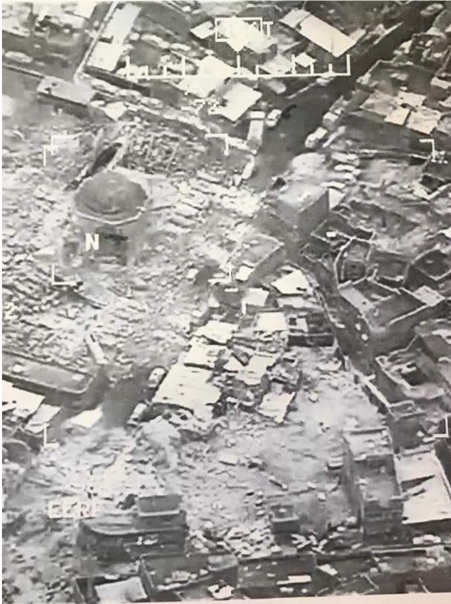
Damage to the al-Nuri al-Kabir Mosque (Iraqi Spring Media; June 21, 2017)
