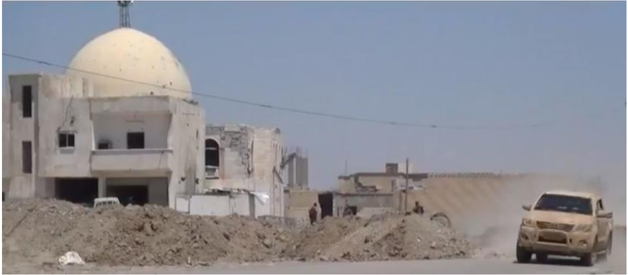
Video still showing damage to al-Subaiha Mosque (RT; June 22, 2017)
