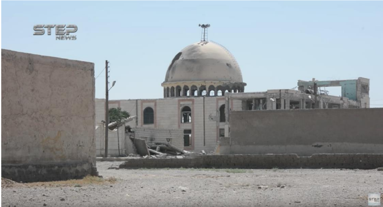
Video still showing damage to al-Subaiha Mosque (Step News Agency; June 12, 2017)
