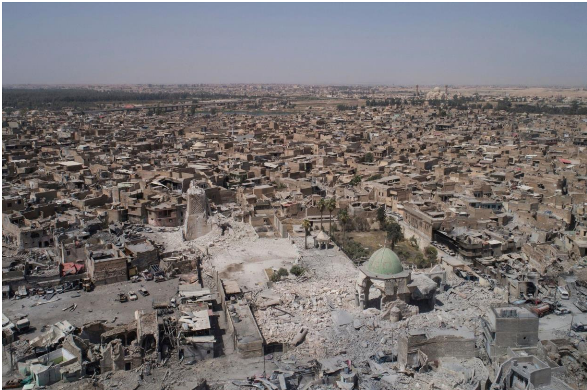
Damage to al-Nuri al-Kabir Mosque, al-Hadba Minaret, and surrounding area (NYT; June 29, 2017)
