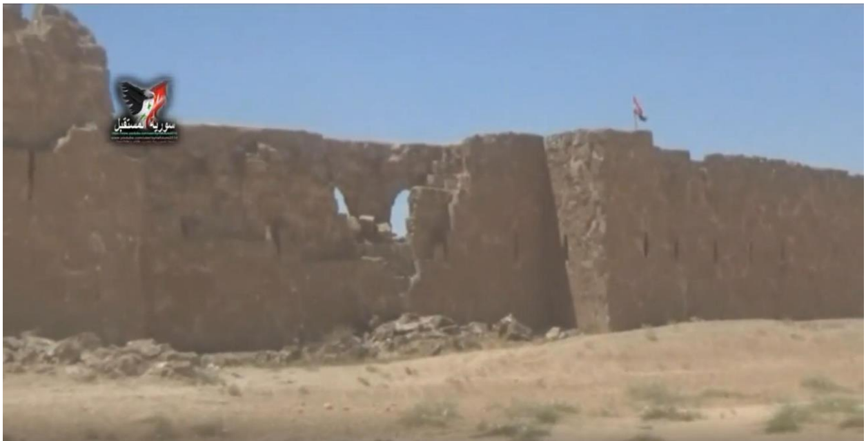
Video still of damage to the city wall of Resafa (Syria al-Mustaqbal; June 21, 2017)
