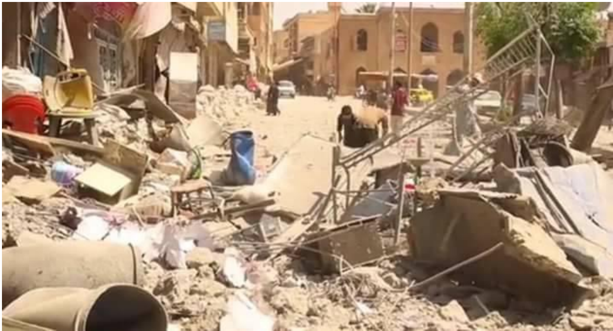
Damage to structures near the Raqqa Museum. The museum is the building with arched windows visible in the top right of the image (Private Facebook Account; June 7, 2017)
