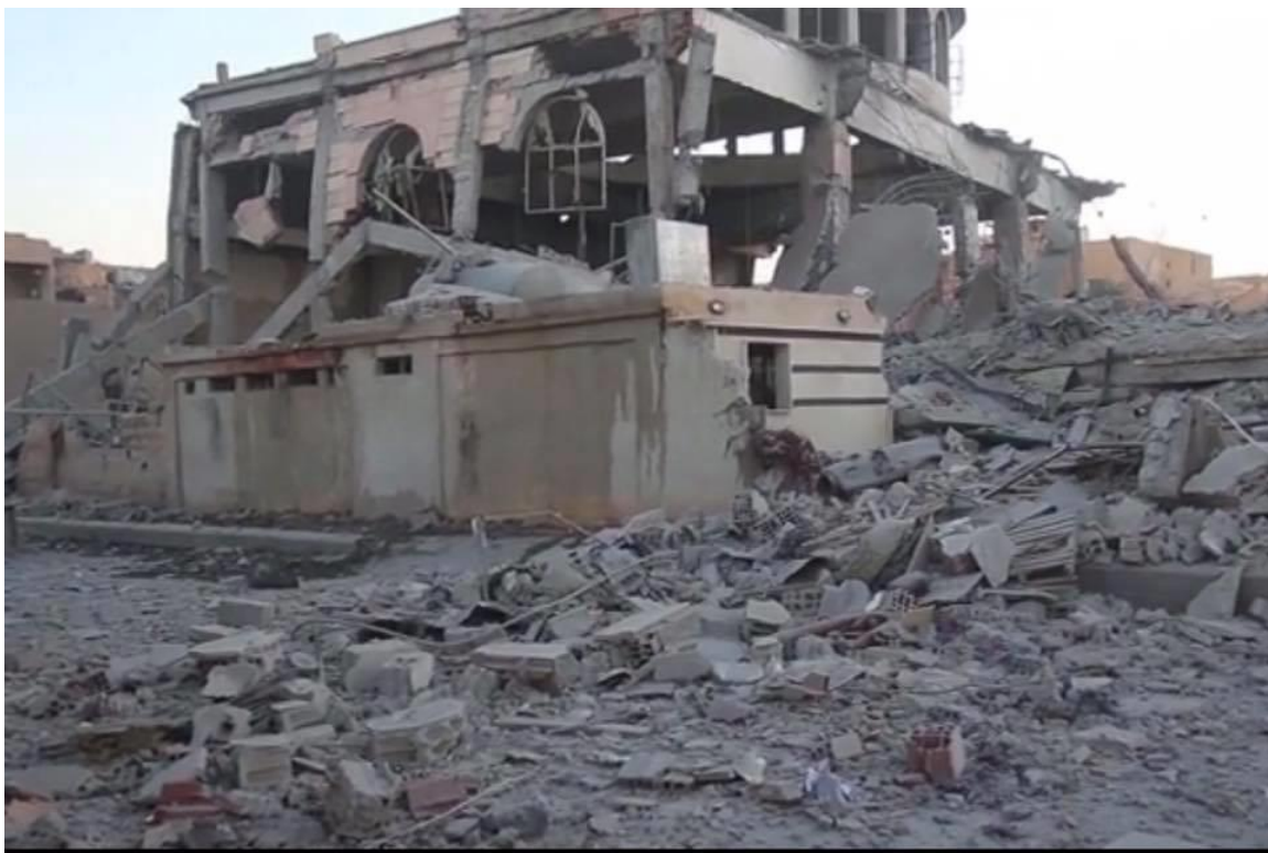
Damage to al-Nur Mosque (RBSS: June 10, 2017)
