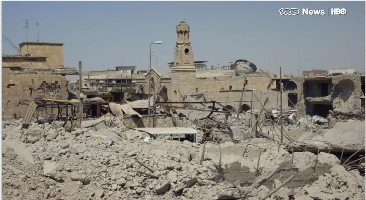
Video still of church showing damage to bell tower and church (Vice News; July 30, 2017)
