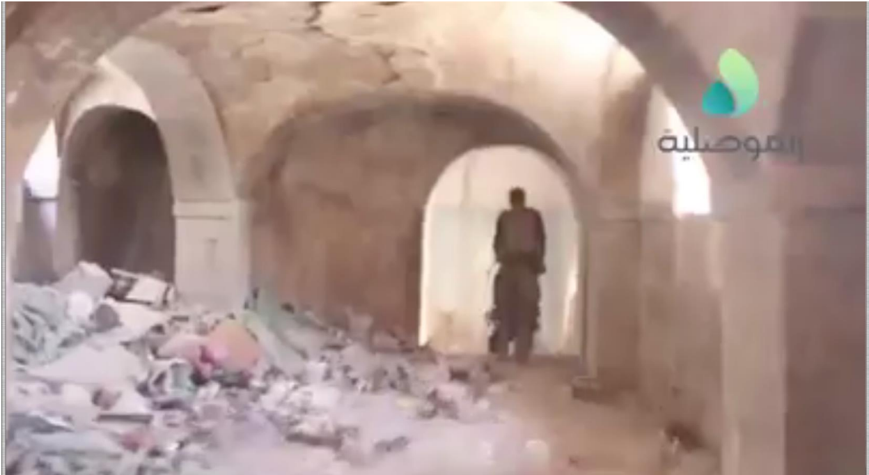
Video still of the interior of Mar Thomas, showing rubble (al-Mosuliya; June 23, 2017)
