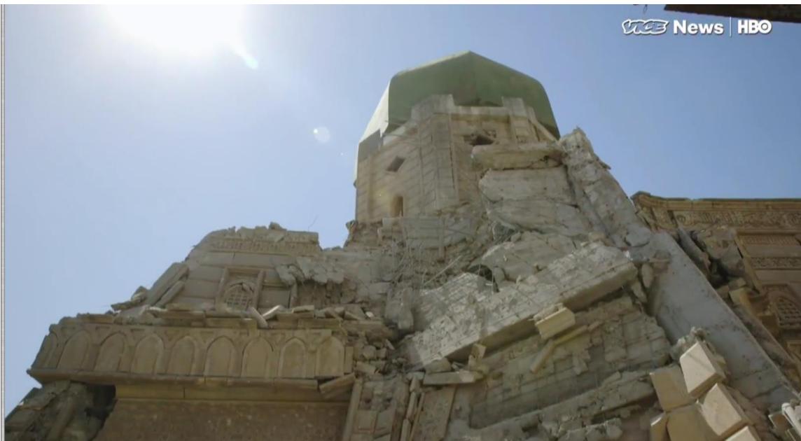
Damage to exterior of al-Imam Muhsin Mosque (Vice News; June 30, 2017)
