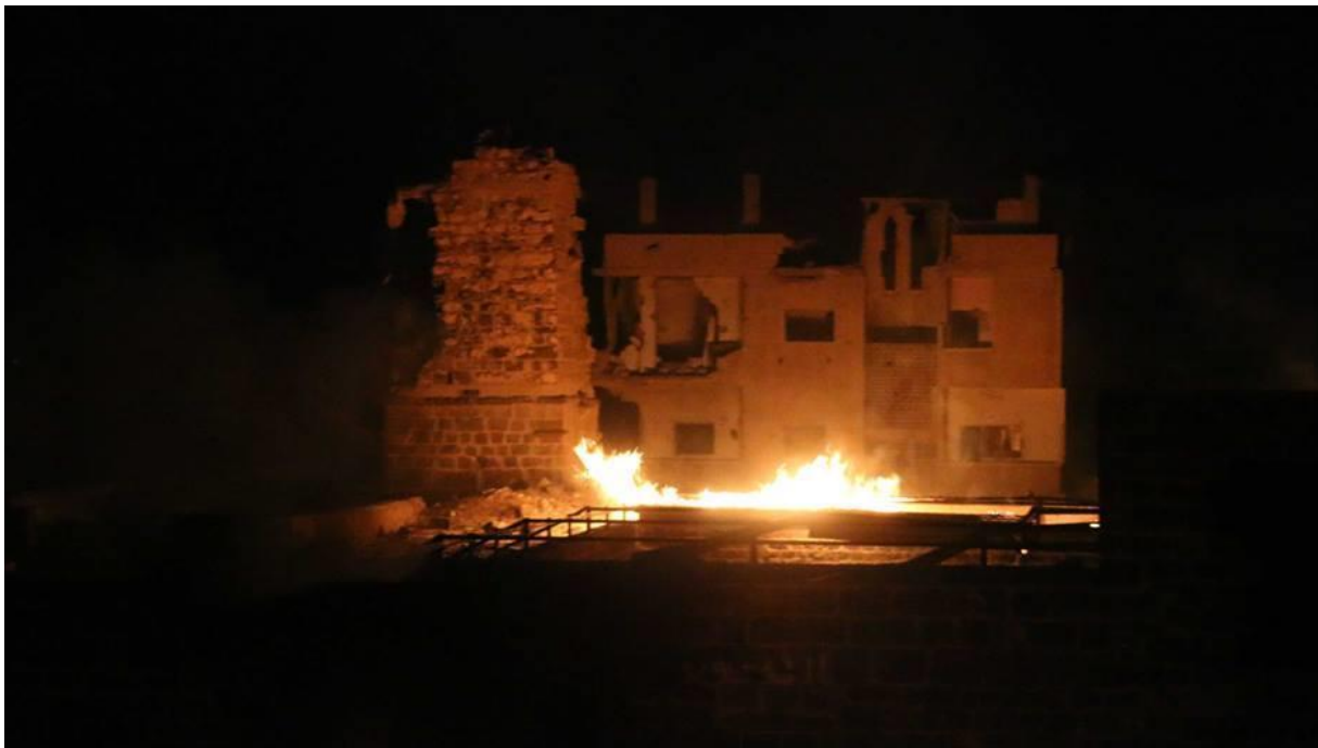
Fires burning inside al-Omari Mosque, the minaret is visible in the upper left portion of the frame (APSA; June 12, 2017)
