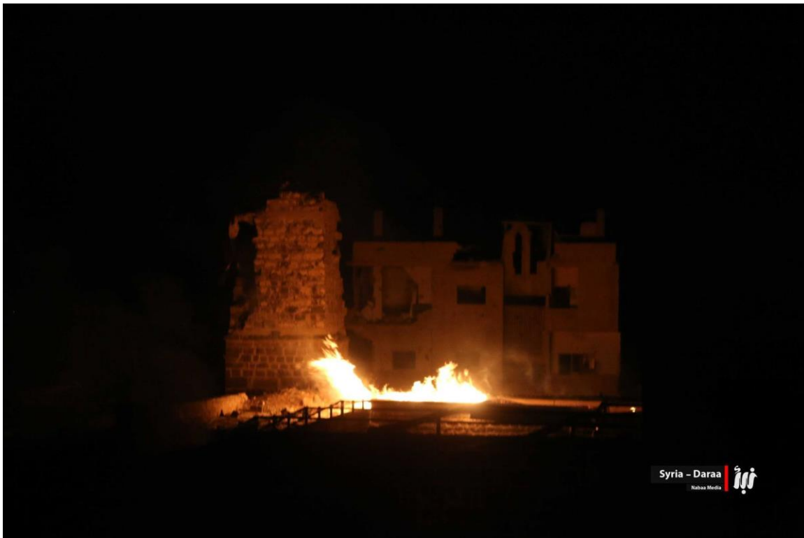
Fire burning inside al-Omari Mosque, the minaret is visible behind the flames. (APSA; June 12, 2017)
