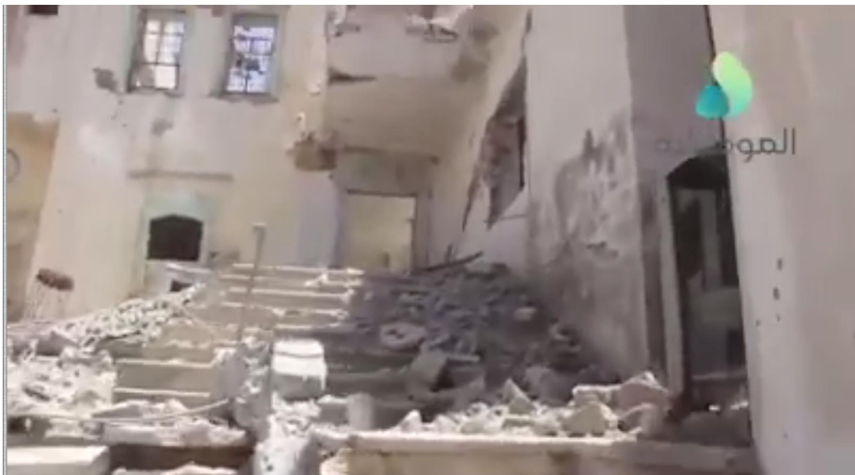
Video still of damage to inside of courtyard (al-Mosuliya; June 23, 2017)
