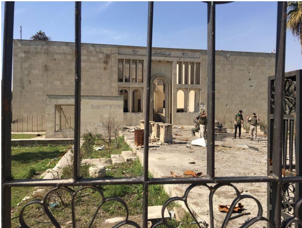
Slight damage to the exterior of the museum, it unknown if this damage is related to recent attack (Personal Facebook Account; June 15, 2017)
