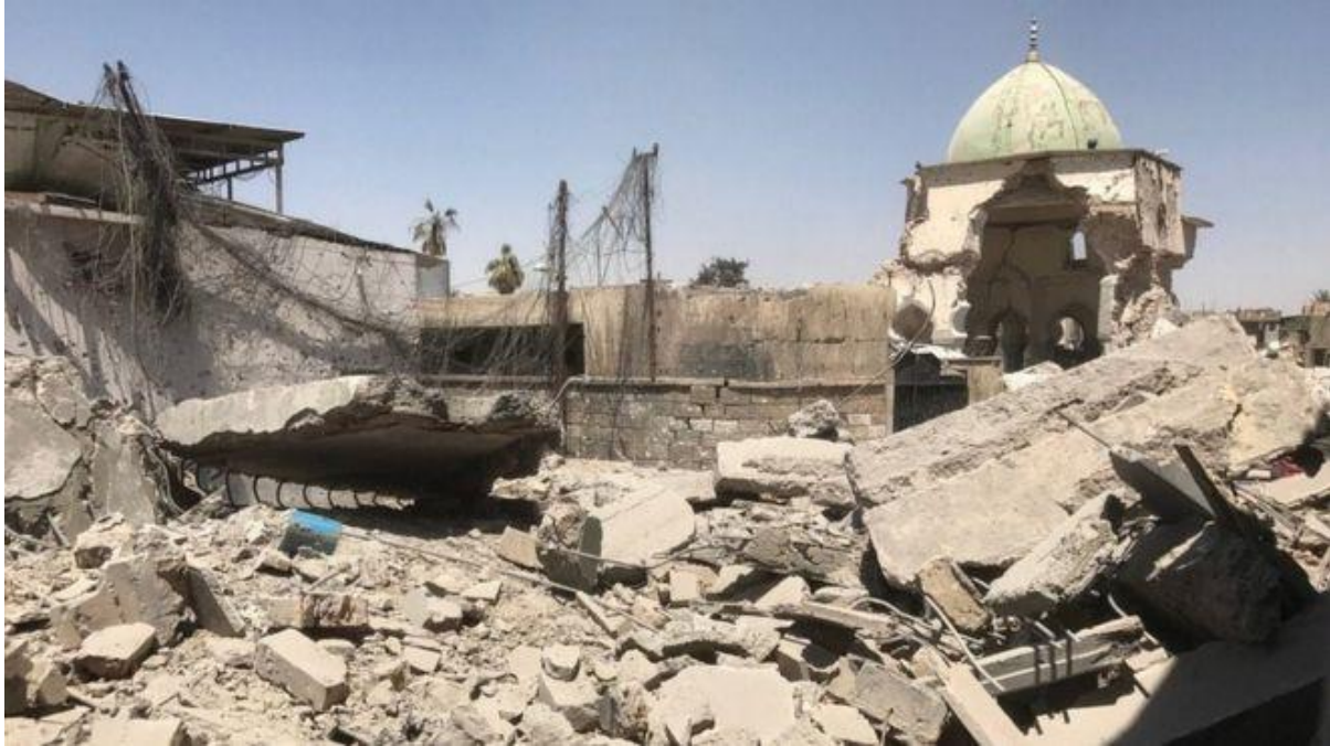
Destruction to al-Nuri al-Kabir Mosque (BBC; June 29, 2017)
