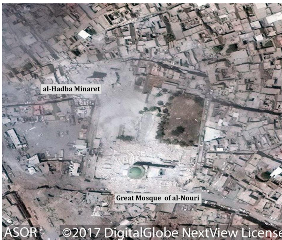
Mosque and Minaret after destruction with the dome still standing (DigitalGlobe NextView License; June 22, 2017)
