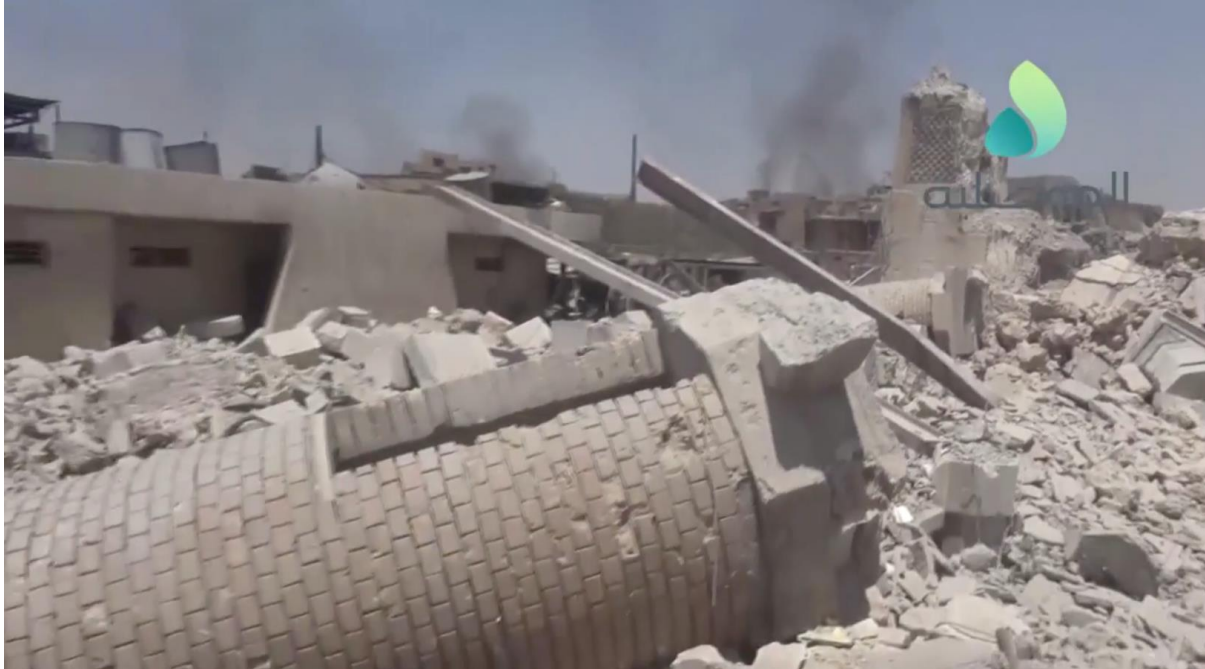
Damage to the al-Hadba minaret showing parts of a secondary minarets on the ground (Al Mosuliya; June 30, 2017)
