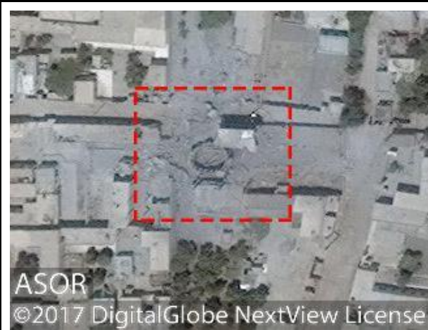
Mosque with severe damage (DigitalGlobe NextView License; June 11, 2017)
