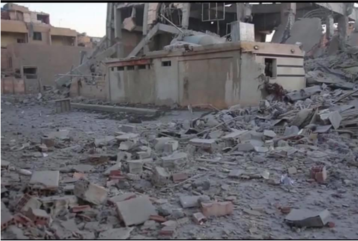
Damage to al-Nur Mosque (RBSS: June 10, 2017)
