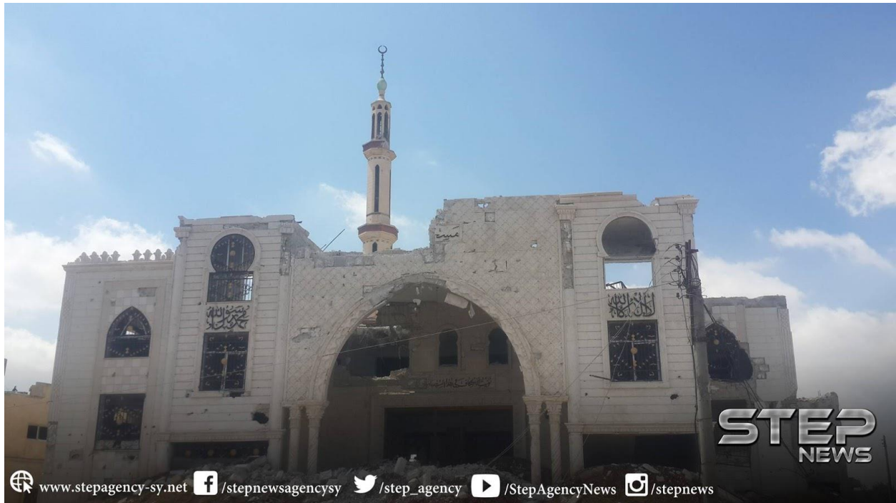
Damage to al-Rahman Mosque, seen from the north (Step News Agency; June 20, 2017)
