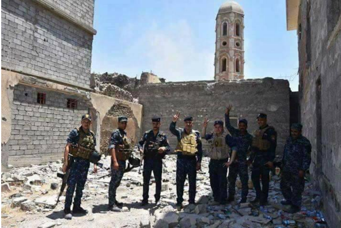
Condition of church today: bell tower still standing, rest of church missing walls (This is Christian Iraq; June 29, 2017)
