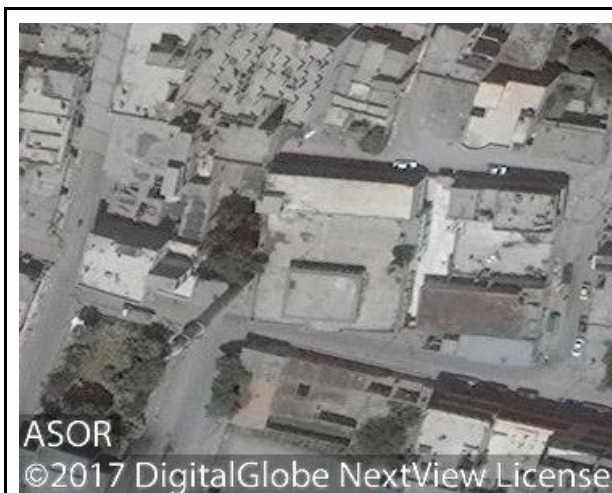
The mosque prior to damage (DigitalGlobe NextView License; June 11, 2017)
