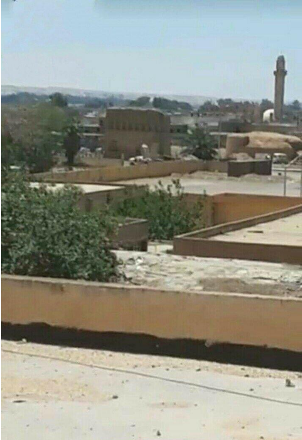
Current condition of Bab Baghdad (Raqqqa Post; June 12, 2017)
