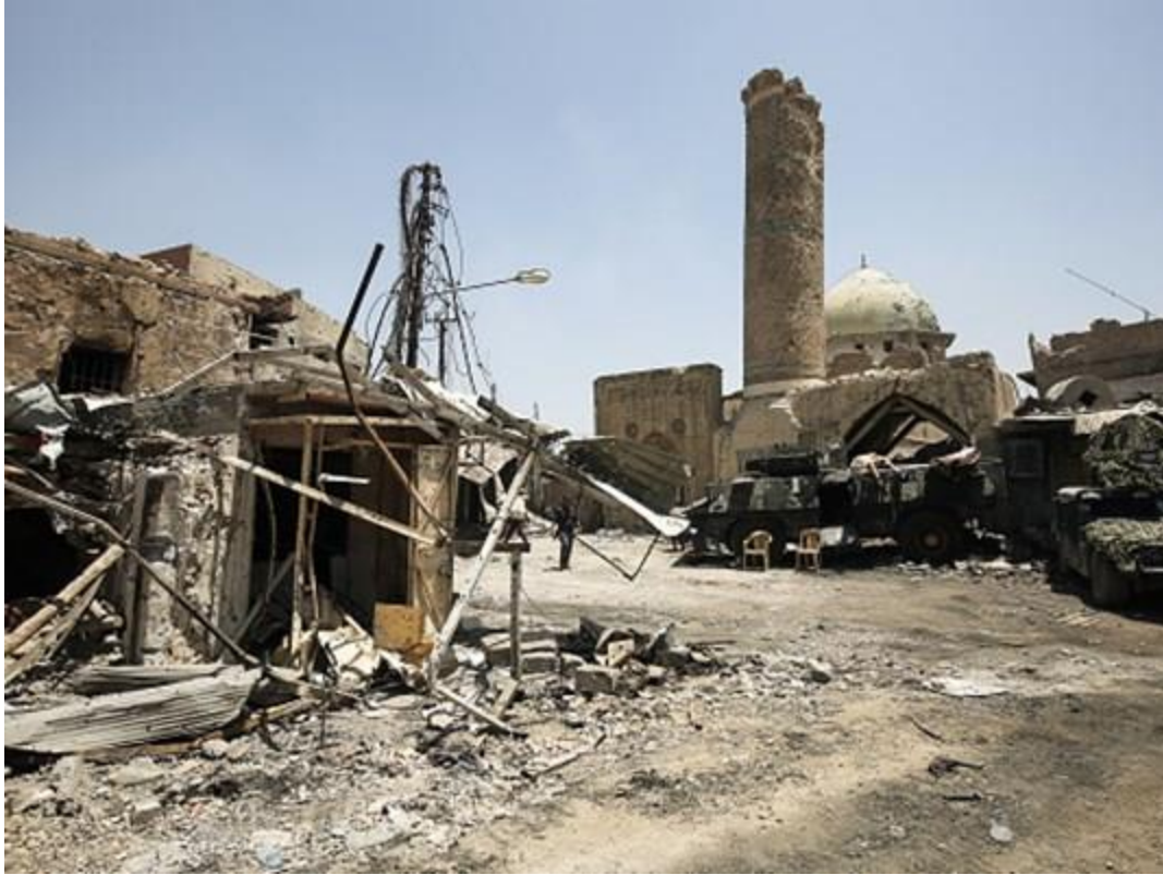
Damage seen to al-Zewani Mosque (AP/WKYC; June 28, 2017)
