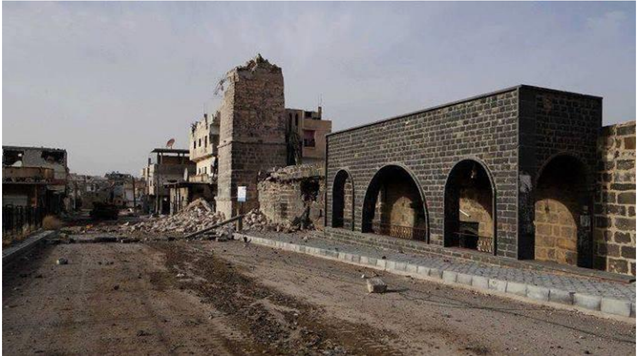
Damage to the minaret and the western side of the mosque. Photograph possibly taken at an earlier date than those featured below (APSA; June 12, 2017)
